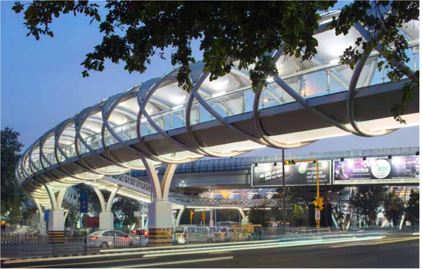
The ITO Skywalk solves the problem of pedestrian movement at one of the busiest nodes in New Delhi, and its unique form is a design and engineering marvel that acts as a significant landmark in the city.
