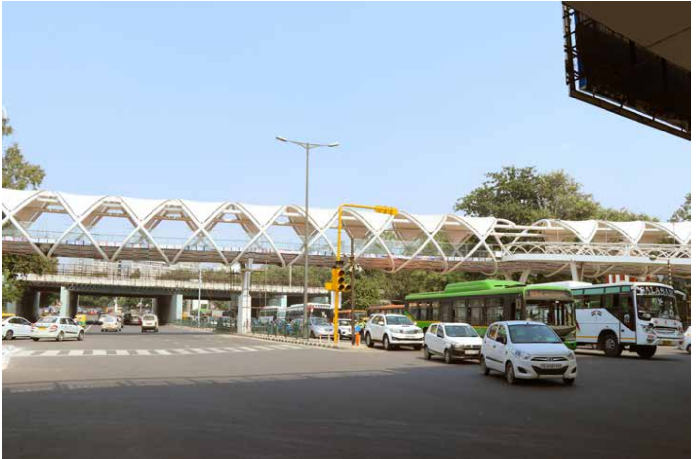
The unique criss-cross boot-lace trusses make the skywalk instantly recognisable from a distance.
