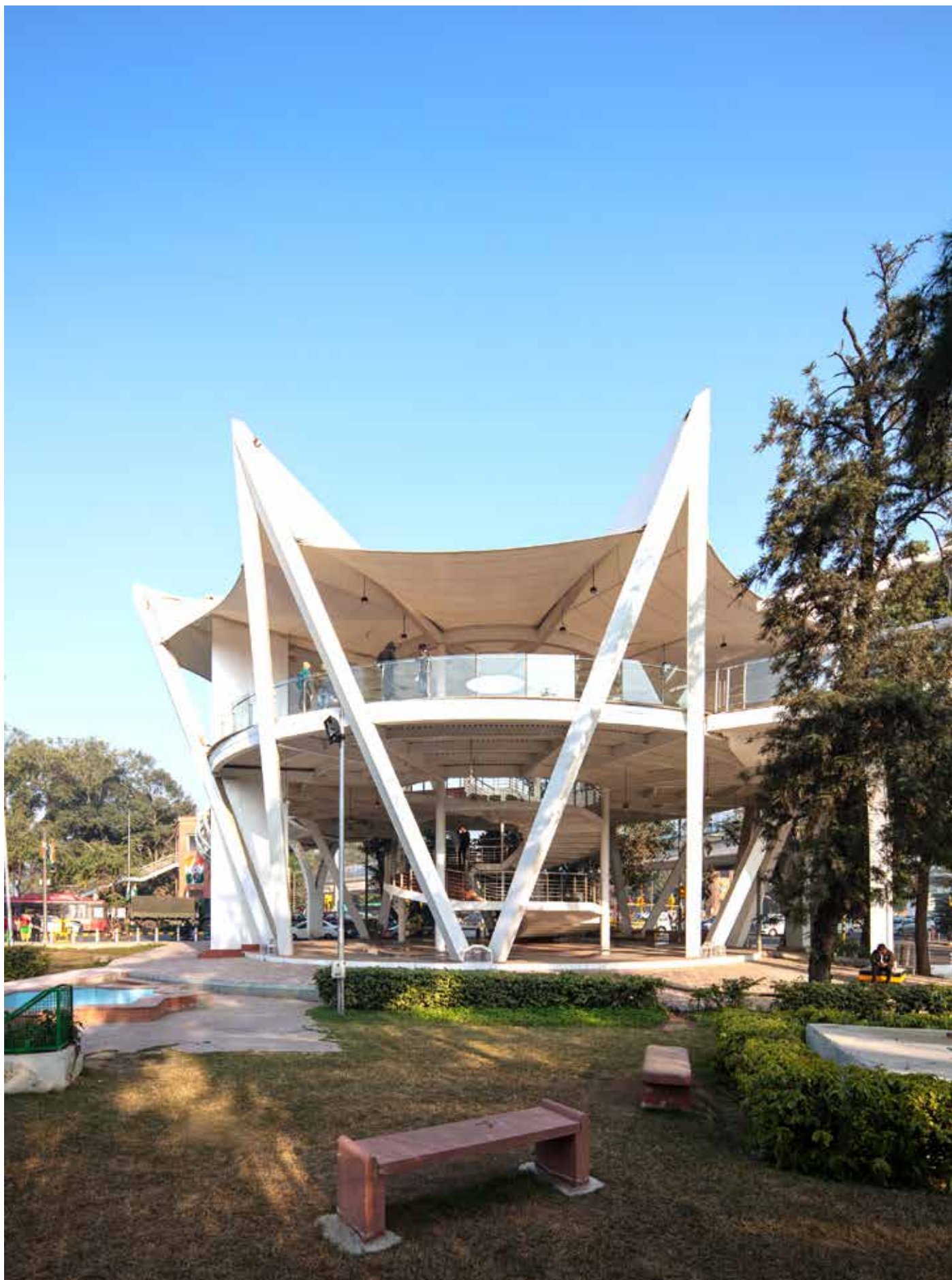
The octagonal unit consists of steel crowns and uses granite flooring and S.S. glass in the railing.
