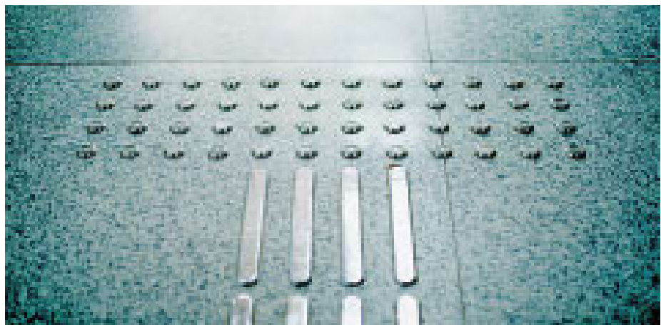
For the visually impaired, facilities include tactile, flooring, tactile railings and low volume audio guidance using PA System.
